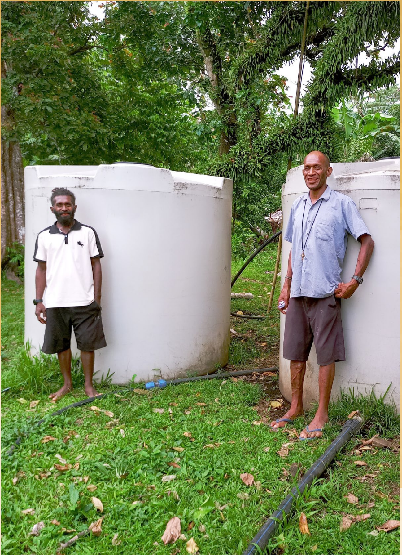
Image: Keithson (L) and Fr Andrew standing with tanks which provide clean water to the health centre and the church at Lavonda-Kairue, Vanuatu. ©Terry Russell, ABM
