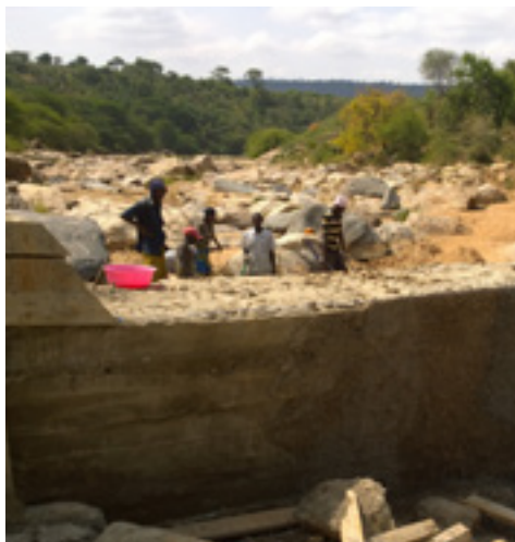
Makakya CBO members work with a mason to construct a sand dam. © Julianne Stewart/ABM 2014.
